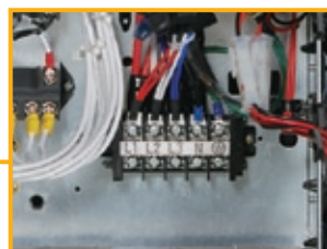
Outdoor unit power supply terminal block
